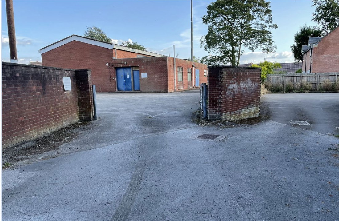
Commercial Premises to rear of site off Private access drive
