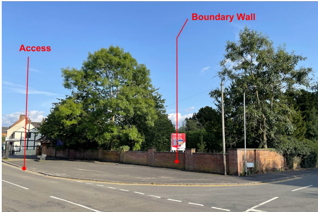
Picture from High Street to Northern Boundary of Site, showing old access point
