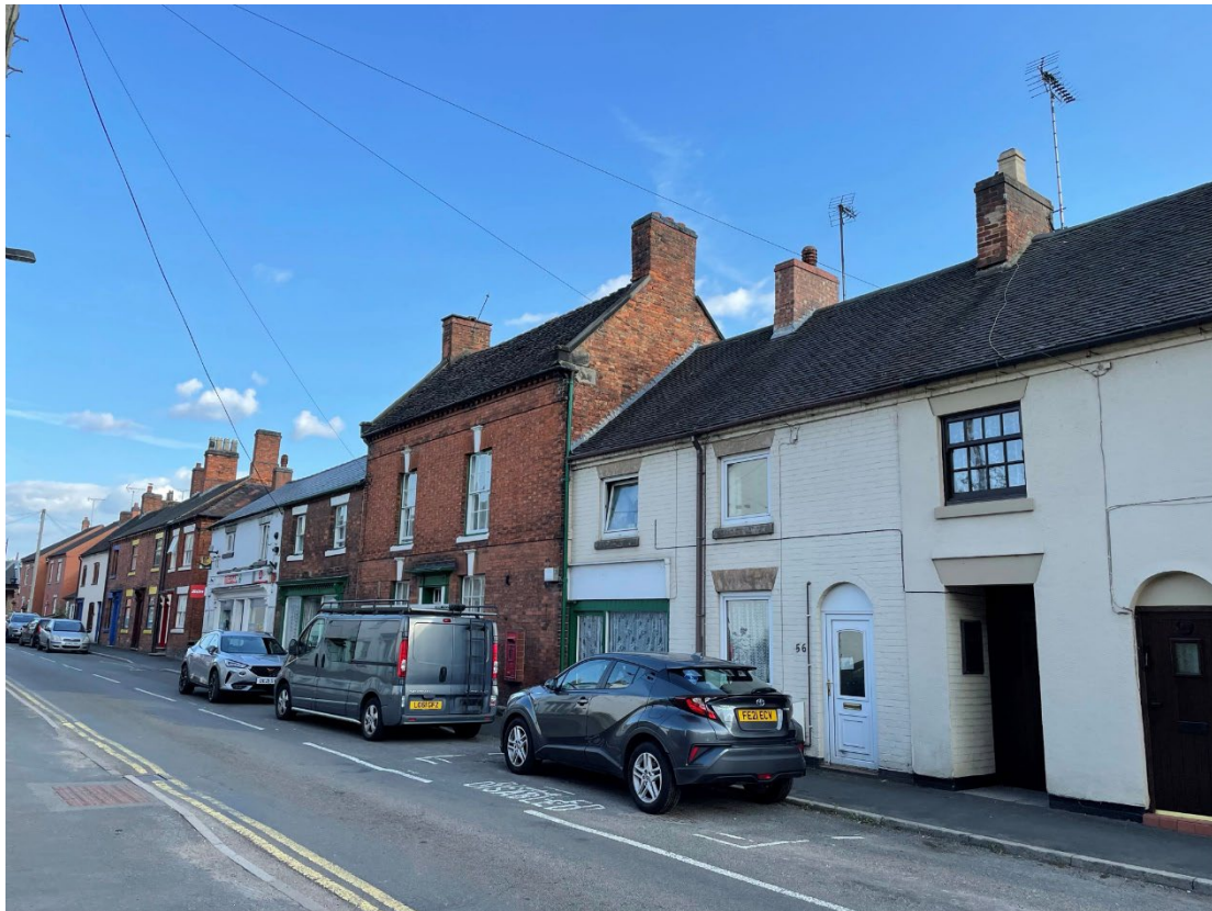
Southern side of High Street
